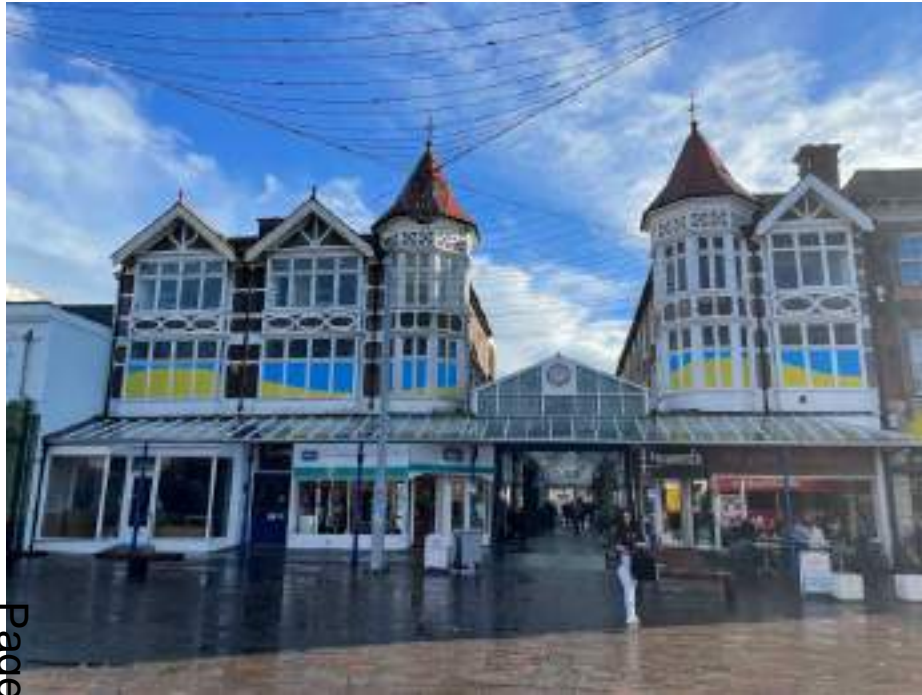
The Arcade, High Street entrance
